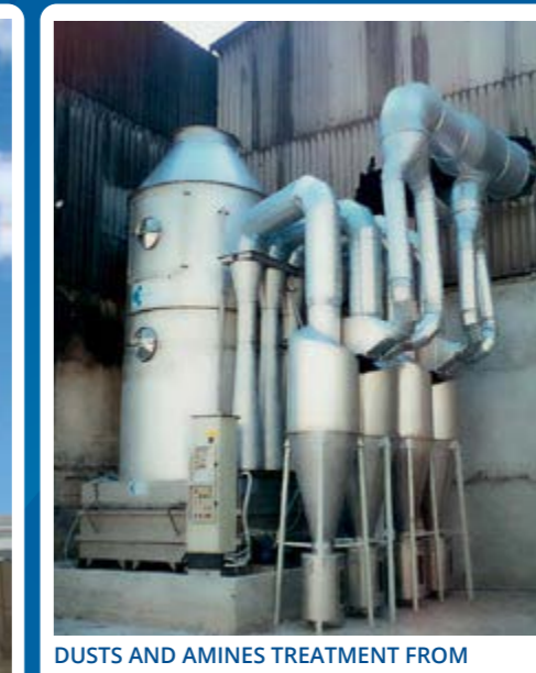
DUSTS AND AMINES TREATMENT FROM COLD-BOX CORE-SHOP DEPARTMENT ABBATTIMENTO POLVERI E AMMINE DA REPARTO ANIMISTERIA COLD-BOX
