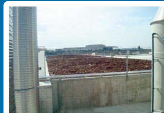
BIOFILTER FOR COV TREATMENT FROM, FOR EXAMPLE, CORE-SHOP DEPARTMENT, POST-CASTING, CORES PAINTING BIOFILTRO PER ABBATTIMENTO COV DA, AD ESEMPIO, REPARTO ANIMISTERIA, POST-COLATA, VERNICIATURA ANIME
