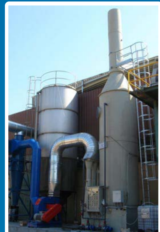
DUSTS, PHENOL AND FORMALDEHYDE TREATMENT FROM SHELL-MOULDING CORE-SHOP DEPARTMENT ABBATTIMENTO POLVERI, FENOLO, FORMALDEIDE DA REPARTO ANIMISTERIA SHELL-MOULDING
